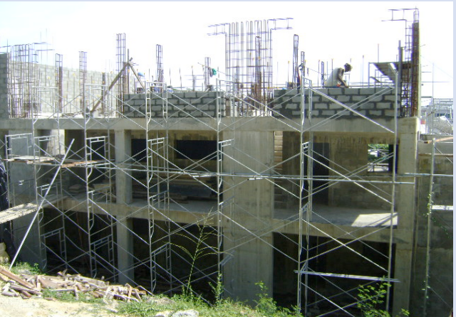
Executive Apartments under construction
