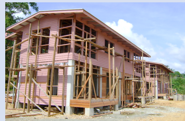
Duplex units at Tasahe under construction
