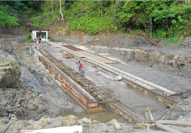
Sasape International Shipyard – under refurbishment and expansion
